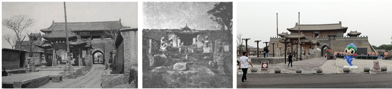
Fig. 1 Yanghe Tower, photos. Left: 1933 (Source: Liang 1933); Middle: 1951 (Source: Liu 1951); Right: 2021 (Source: the author)
